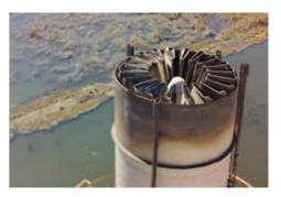
An image of a flare tip taken by a drone.
