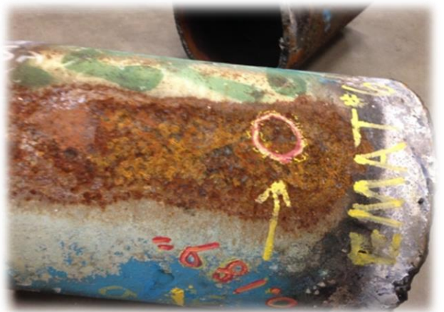
IRISNDT estimated 40% cross-sectional wall loss Follow-up results: 43% wall loss
