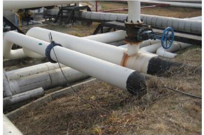
An overview of the pipe at the earth penetration
