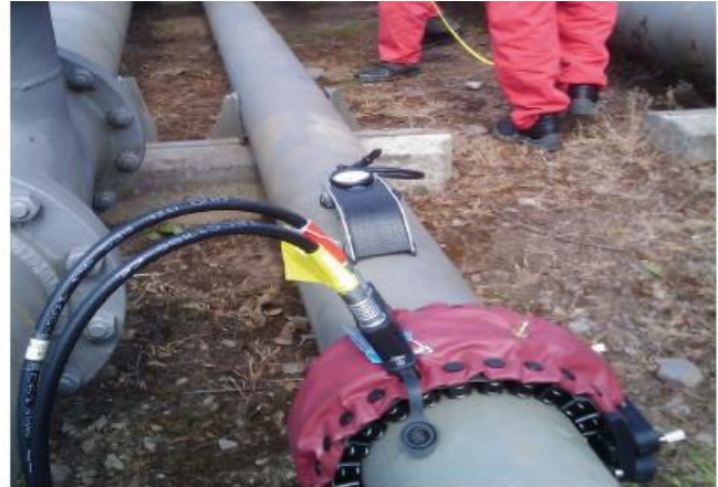
The view of the test pipe in the backward direction.
