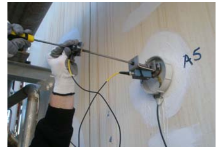
Waveguide Screwed to a Coupling on a Double-Walled Tank
