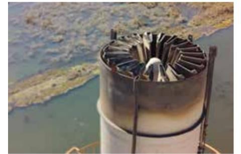
An image of a flare tip taken by a drone.
