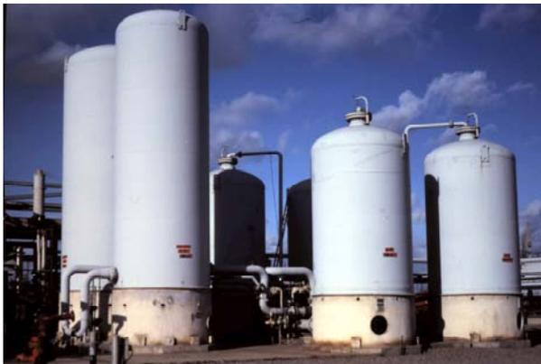
In the case of new vessels, the stimulus for AE activity is from the standard hydrotest. This type of test can detect weld defects and localized yielding at hydrotest pressures, especially in non-stress relieved vessels.
