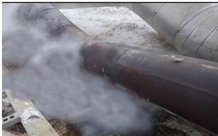
Figure 1 – Steam Leak in Above Ground Steam Pipeline
